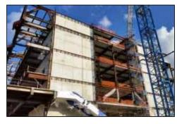
View of NW corner core and escalator, with cantilevered floor extensions.
